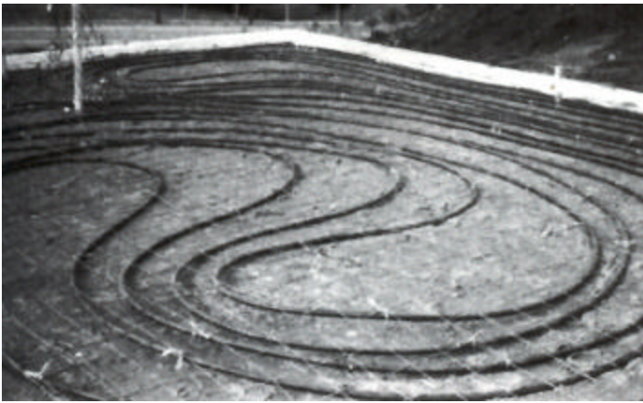
Four 220-ft lengths of 0.75"-ID high-density polyethylene tubing are imbedded in the 5.5" thick slab-on-grade of the test house. Beneath the slab, 600-ft. of tubing runs through a 2-ft layer of gravel.
