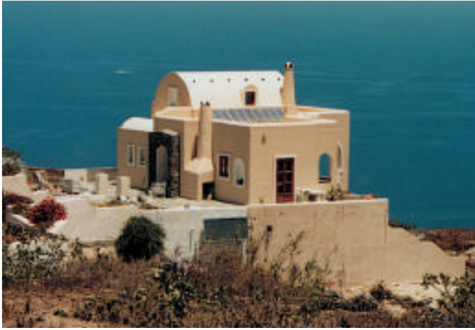
A more contemporary Greek home on San torini uses masonry construction and makes good use of the sun.
