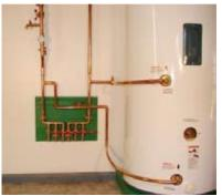
Note: Plan to avoid over heating at plastic fittings. The solar collector antifreeze loop can get very hot if it is only making domestic hot water. Make sure that heat cannot conduct to plastic fittings or other components that are not rated for high heat. The tubing that connects to the solar domestic tank can get very hot. Provide 18 inches of uninsulated vertical separation between the solar tubing and any plastic connections at the supplements manifold.
