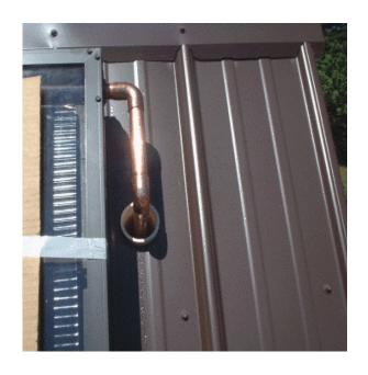
b. Compatible Materials - Whenever possible, use mounting hardware that is supplied by the solar collector manufacturer. It is essential to avoid the use of different kinds of metals when fastening to the solar collectors. When different kinds of metals are used, the metal that is more stable will corrode the metal that is less stable. Use stainless steel fasteners, which are especially resistant to corrosion, or use components that are all made of the same material.
