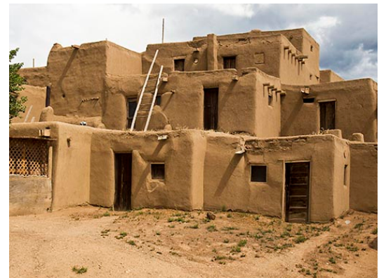
The Pueblo and Anasazi Indians faced their buildings directly south and used material that would store heat and cool temperatures.
