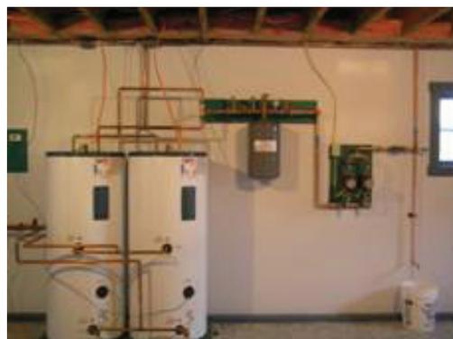
The testing facility was constructed of typical frame construction and was divided roughly in half in order to observe different tubing strategies under equal and identical conditions and make meaningful comparisons between the two without the issues of confounding variables. Heating performance is determined by very careful measurements of water flow and temperature measurements of the water going into and out of the systems.
